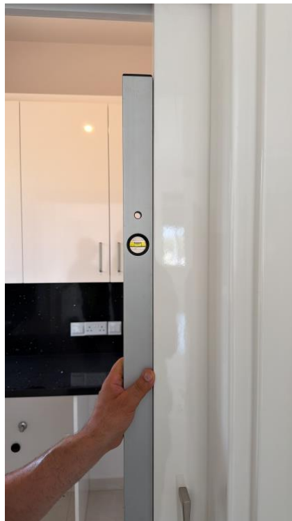
Figure 26. Alignment check to the sliding-door frame.
