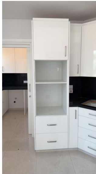
Figure 30. Overall view of the kitchen joinery installation.
