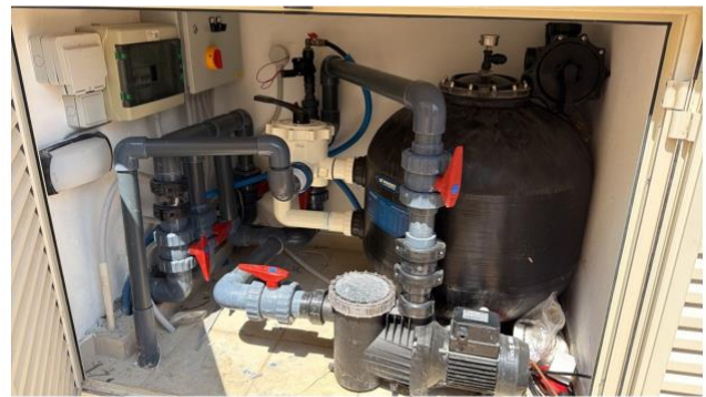
Figure 18. Overall view of the pool plant and associated pipework.
