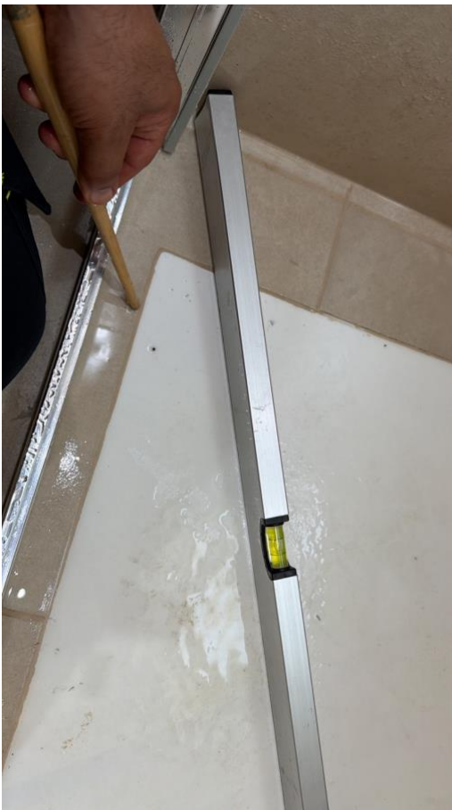
Figure 42. Level check to the master-bathroom shower floor finish.
