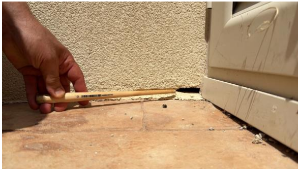
Figure 3. Open external junction capable of admitting water.
