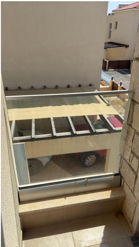
Figure 48. Glass balcony balustrade checked for stability during the inspection.
