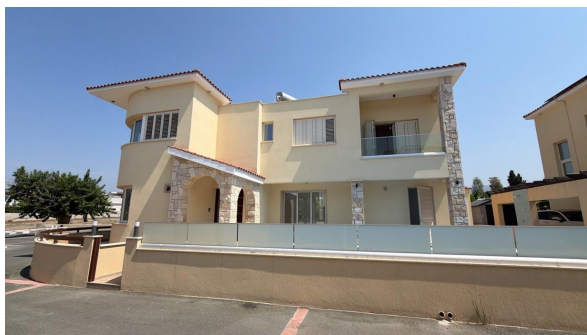
Figure 1. Front elevation of the inspected villa.
