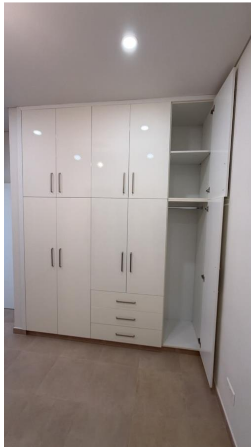
Figure 53. Overall view of the wardrobe installation and affected door.
