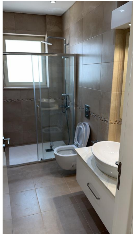
Figure 43. Overall view of the master-bathroom shower area inspected for drainage and falls.
