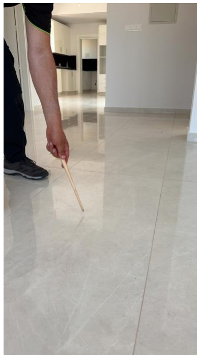
Figure 23. Additional ground-floor tile location checked by tap testing.
