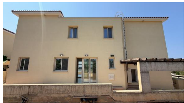
Figure 2. Rear elevation and roof-access ladder.
