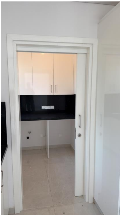
Figure 25. Overall view of the kitchen internal sliding-door opening.
